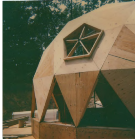
The struts on my dome are 5 foot three, six foot three
