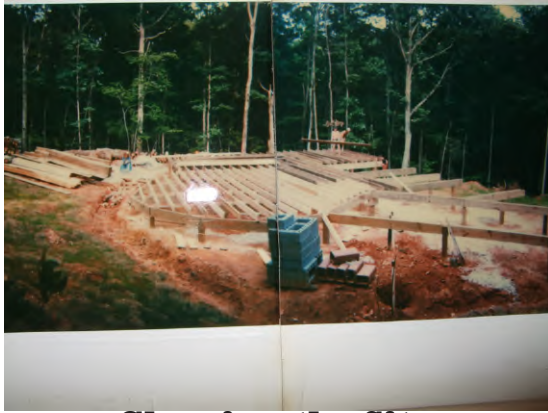
Clearing the Site
